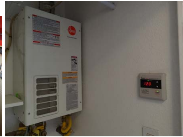
Rheem tankless always on water heater for residential side
