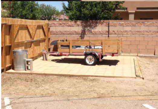
Trailer pad and two large gates provide access to Keleher Avenue, from backyard
